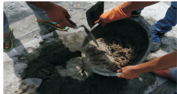
Figure 6. Pouring of modified Jute Cement slurry in Sand-cement Mix
